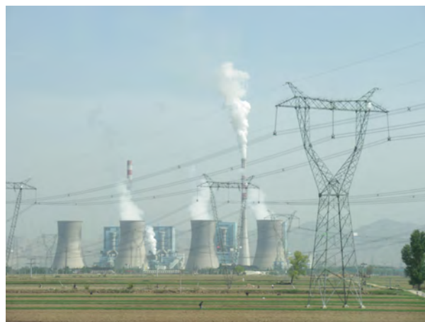
FIGURE 7.22 Tremendous amounts of electric power are generated by coal-fired power plants such as this one in China, but an even larger amount of power goes into heat transfer to the surroundings. The large cooling towers here are needed to transfer heat as rapidly as it is produced. The transfer of heat is not unique to coal plants but is an unavoidable consequence of generating electric power from any fuel—nuclear, coal, oil, natural gas, or the like. (credit: Kleinolive, Wikimedia Commons)
