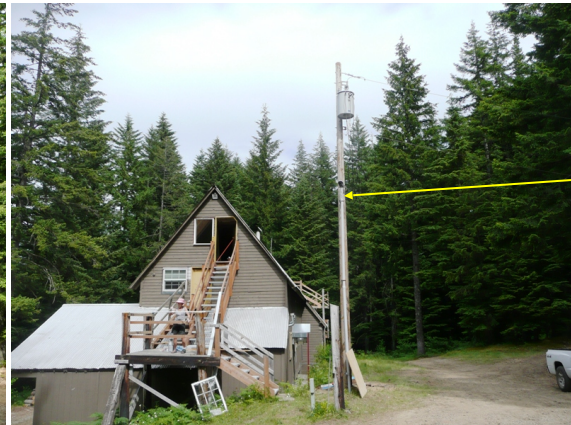
New pole at the Lodge
