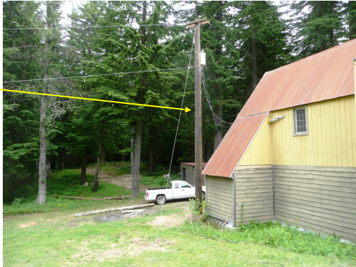
New pole at Tow Hut
