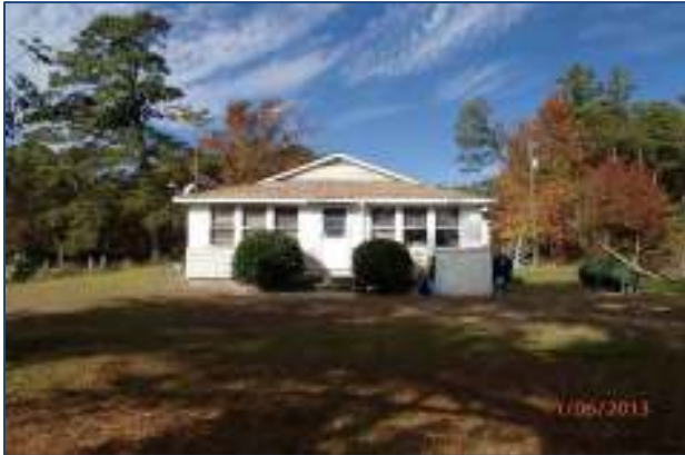
Figure 77: House in Hayes, Gloucester County - BEFORE elevation.
