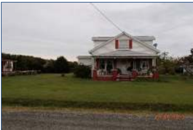
Figure 79: House in Hayes, Gloucester County - BEFORE elevation.
