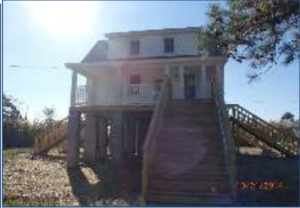
Figure 76: House in Hayes, Gloucester County - AFTER elevation.
