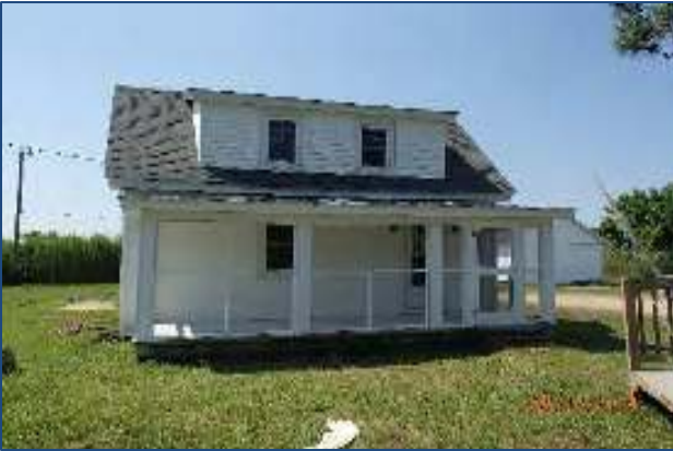
Figure 75: House in Hayes, Gloucester County - BEFORE elevation.
