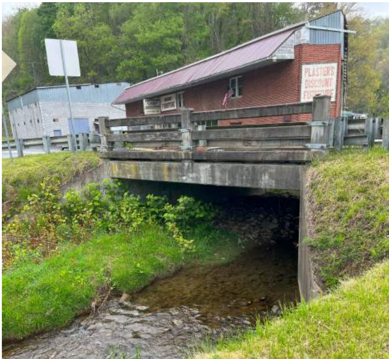
Figure 727: Culvert crossing Mill Creek
