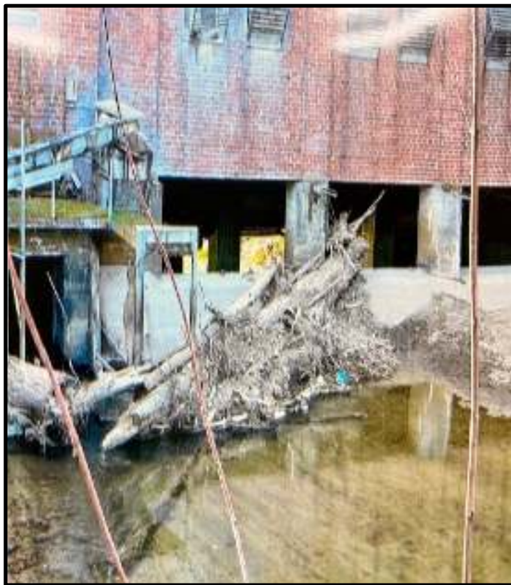
Figure 2. Debris Gathered on Upstream Side of Abandoned Mill Building in the Town of Tazewell
