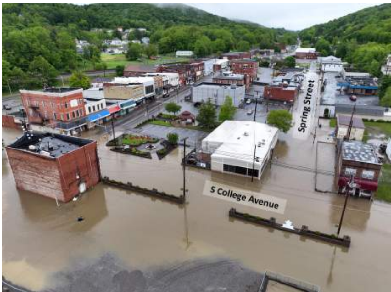
Figure 728: Downtown Bluefield flooding – May 29, 2023
