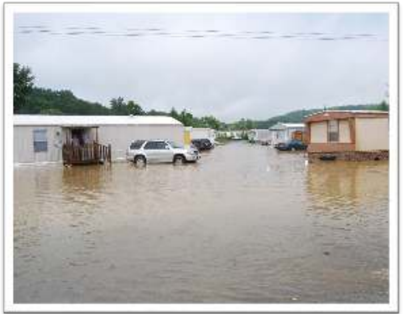
Photo 5: Flooding in C&C Mobile Home Park (2011)
