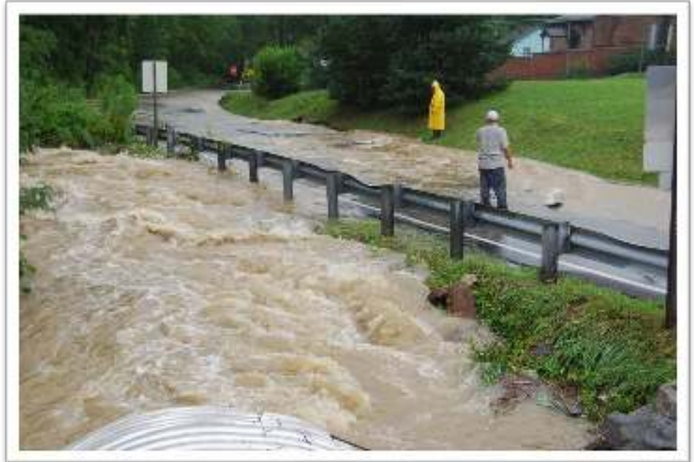
Photo 2: Yellow Creek Road Pavement Buckling (2011)
