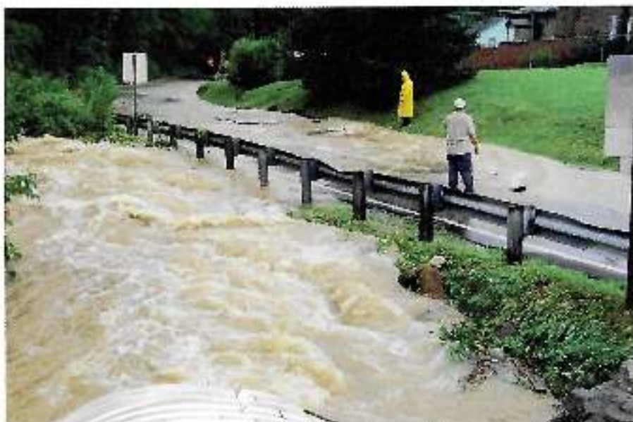
Photo 2: Yellow Creek Road Power out, Flooding (2017)
