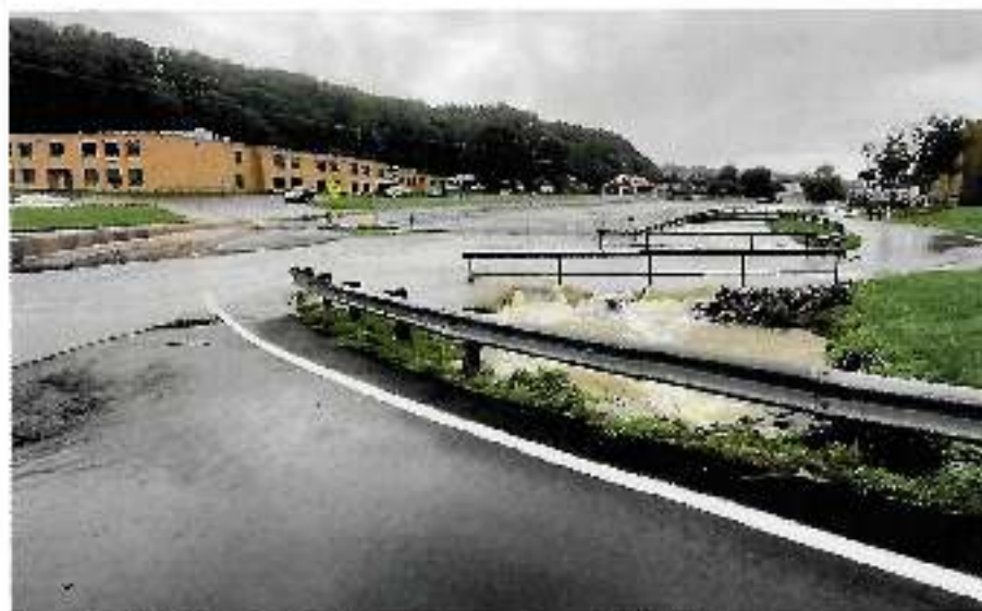
Photo 3: Flood Waters Between I. F. Adair High Middle School and Wise Primary School (2022)
