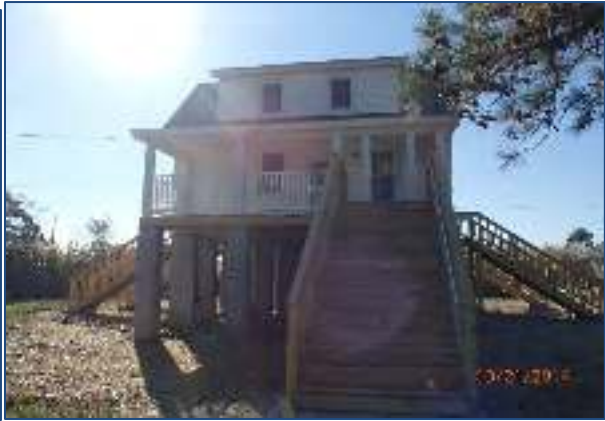
Figure 76: House in Hayes, Gloucester County - AFTER elevation.
