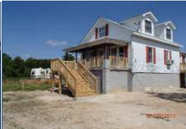
Figure 80: House in Hayes, Gloucester County - AFTER elevation.
