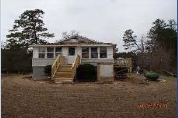
Figure 78: House in Hayes, Gloucester County - AFTER elevation.
