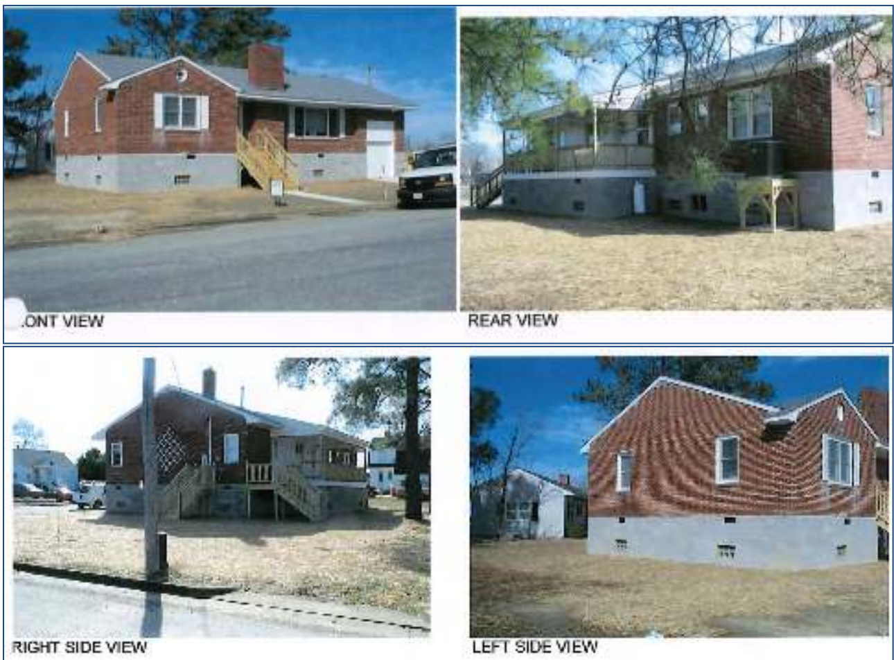
Figure 84: Photos of a home in the Town of West Point after being elevated.
