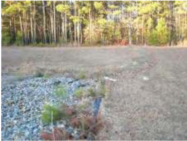
Figure 1: Infiltration trench w/ low earthen berm
