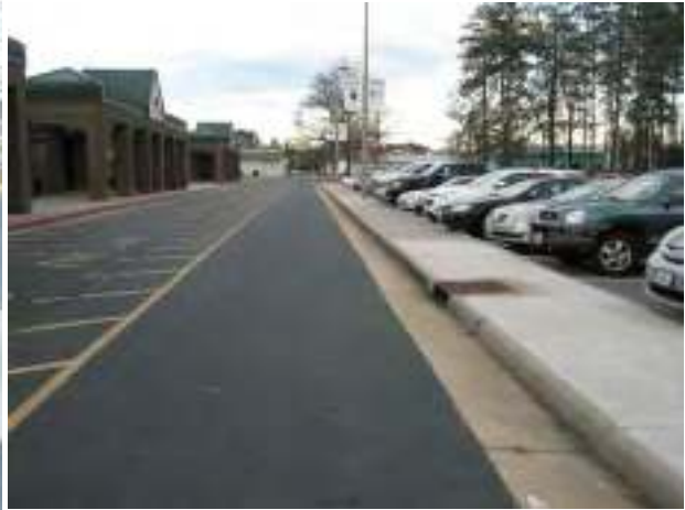
Photo 2: Driveway drainage to Biofilter B
