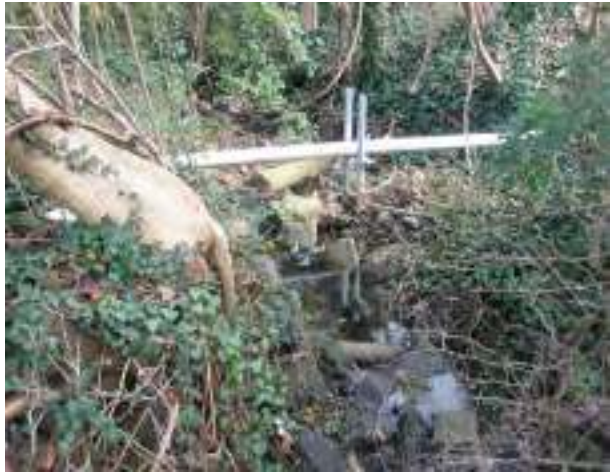
Figure 1: Downstream of existing BMP
