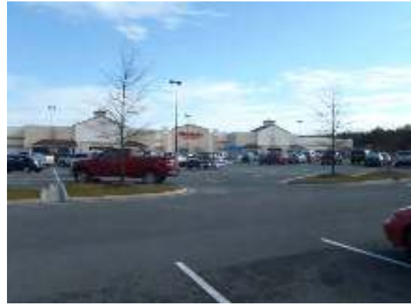
Figure 2: Drainage area leading to potential retrofit
