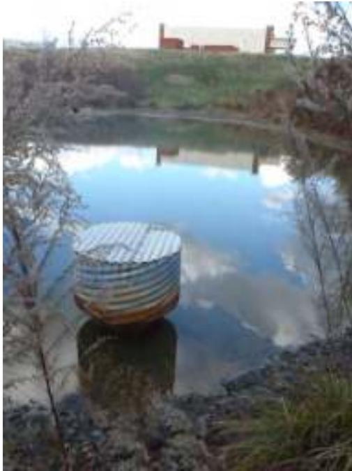
Figure 1: Wet pond with metal overflow structure
