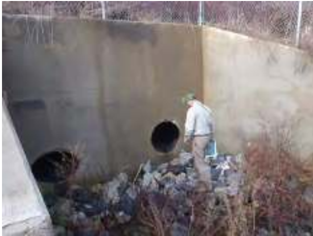
Figure 15: Concrete headwall above S-103
