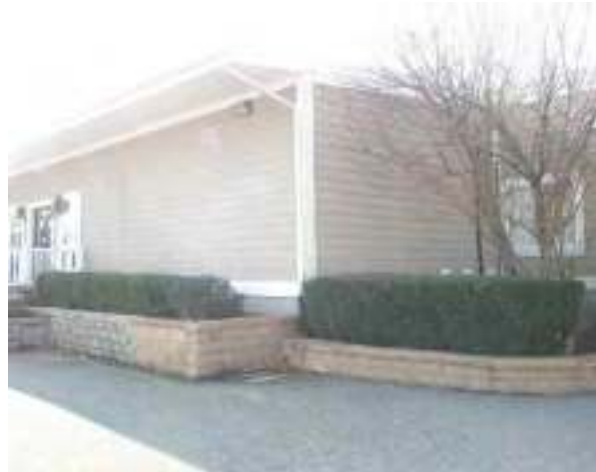
Figure 1: Right side downspout
