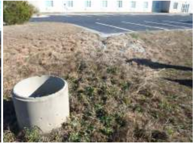
Figure 2: Riser structure at northern end of basin
