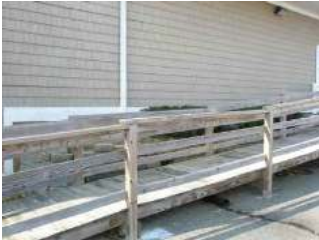
Figure 1: Left side of building downspout
