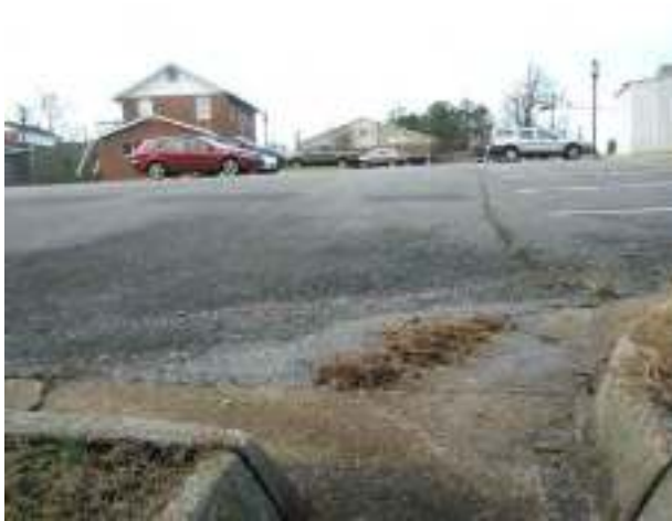
Figure 1: Existing drainage from parking lot
