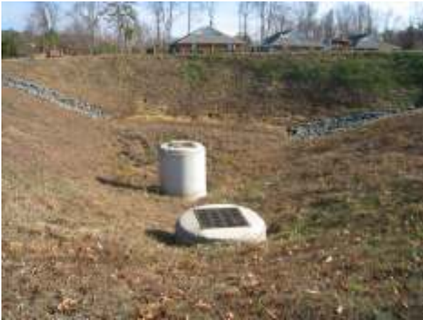
Figure 3. Detention basin in communal area
