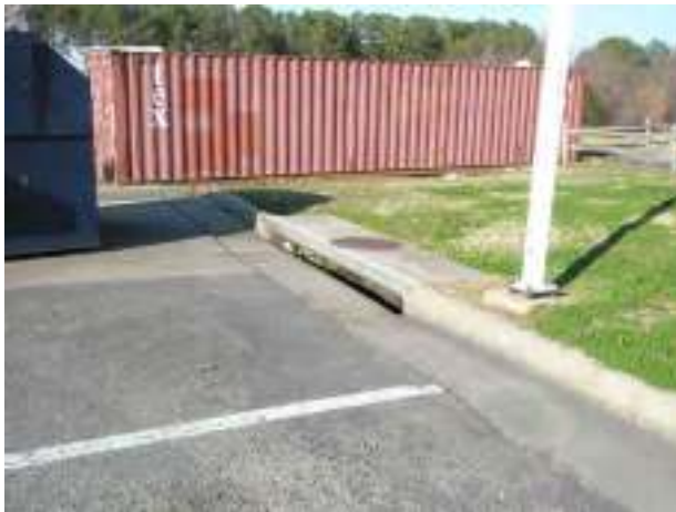
Figure 3: Curb inlet draining 0.8 ac gas station
