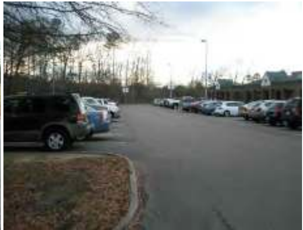
Photo 4: Drainage to Dry Swale/Retention Trench
