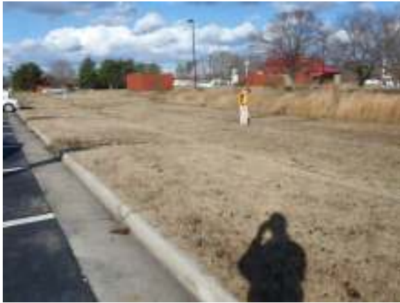
Figure 1: Northern end of detention basin
