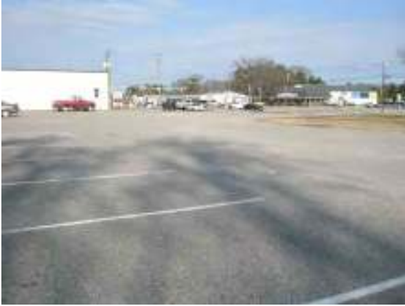
Figure 3: Paved area in front of building
