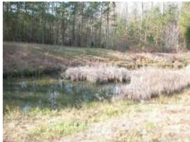
Figure 1: Stormwater basin behind shopping center
