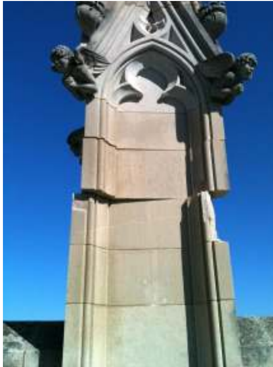
Figure 26: Earthquake Damage to Washington National Cathedral in Washington, D.C. After the 2011 Earthquake 77
