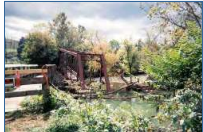
Hurricane Isabel - South River in Rockbridge County
