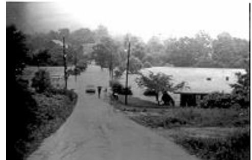
Rising water in Waynesboro from Hurricane Camille.
