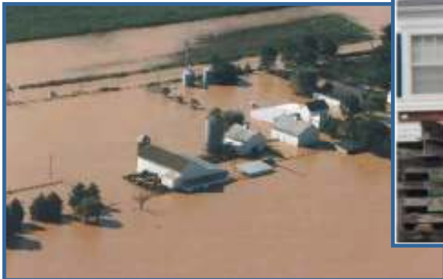
Photo II-1: Flooding in Rockingham County, Hurricane Fran, 1996
