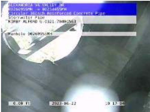
009390STMP_f643a7f3-2f0f-4551-96c3-14cc68e2dded_2023 0622_104954_298.jpg, 00:00:00, 0.00ft Manhole / 002609SSMH
