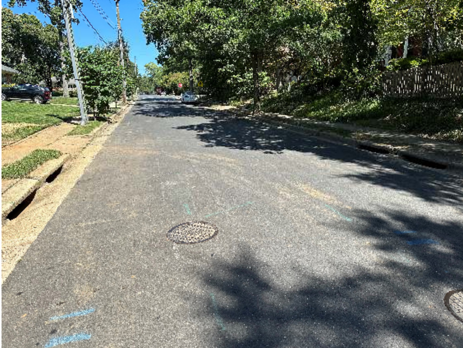
Picture 6 : Dual curb inlets on both sides of Valley Drive between Summit Avenue and Dogwood Drive. Facing north.
