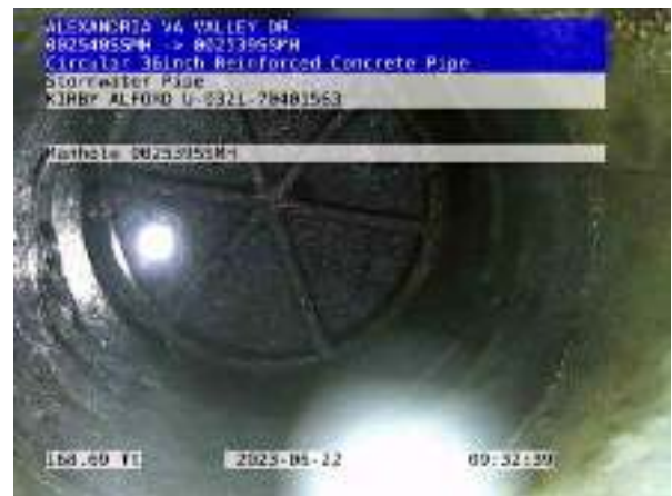
009067STMP_84177e0d-4f74-4694-9cca-08aa6088da47_20230622_100528_417.jpg, 00:03:34, 168.69ft Manhole / 002539SSMH
