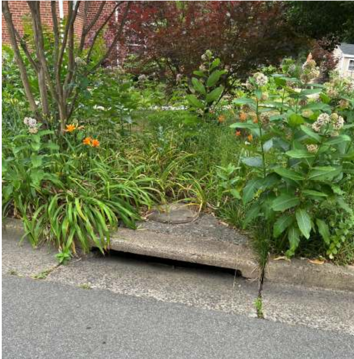
Picture 1 : Storm drain curb inlet 005458IN at the sump near the intersection of Crestwood Drive and Valley Drive, facing south. Approximate inlet dimensions 4"x3.5'.
