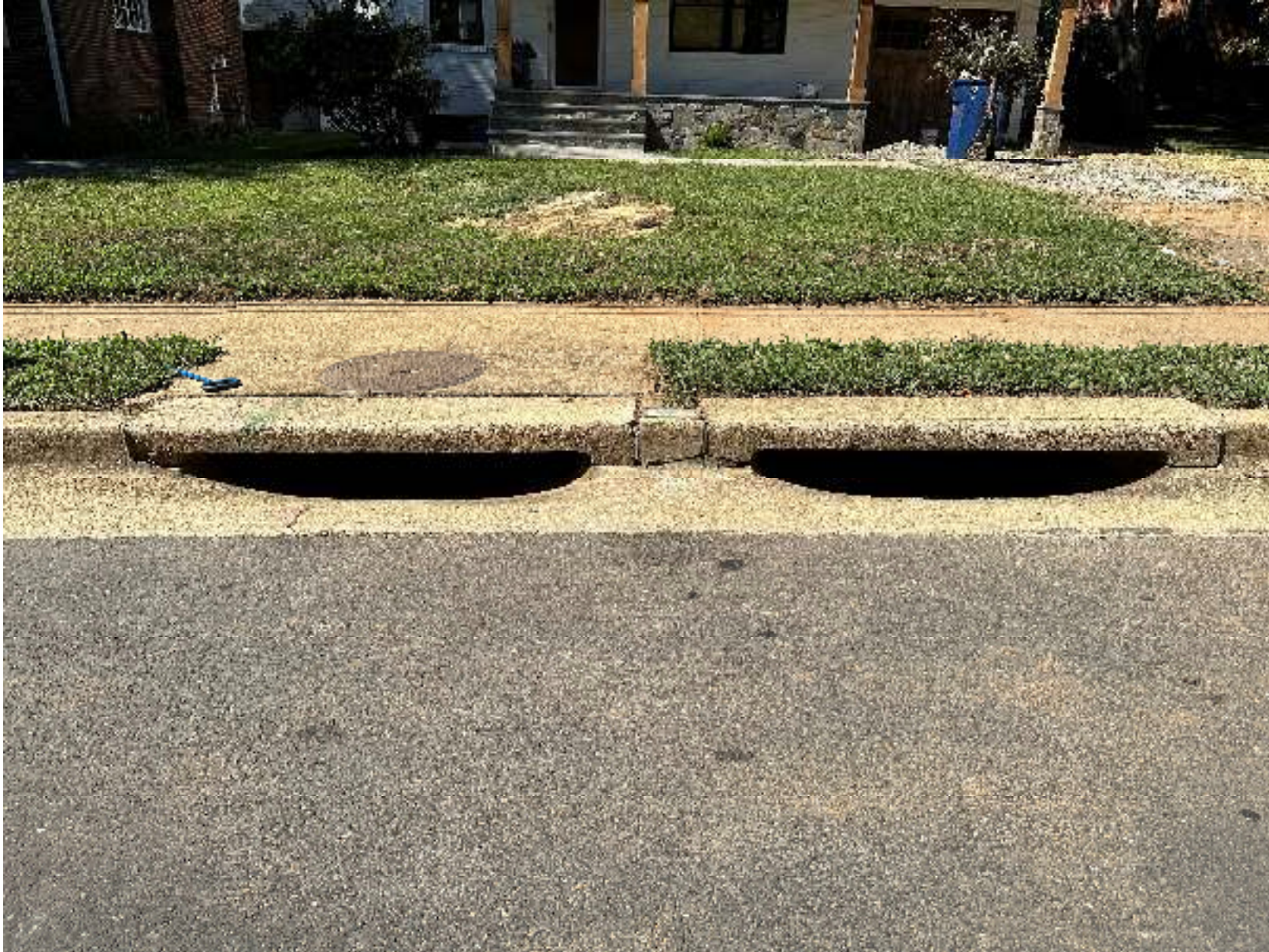
Picture 5 : Curb inlets (005542IN) along the west side of Valley Drive, approximately 2-6"x4'. Facing west.
