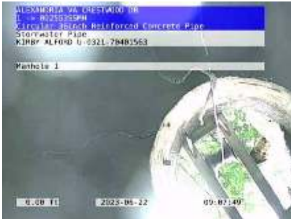
008275STMP_6c49d1a6-4cd3-466f-91a2-6b2be2b9b9ba_20230622_094038_348.jpg, 00:00:00, 0.00ft Manhole / 1
