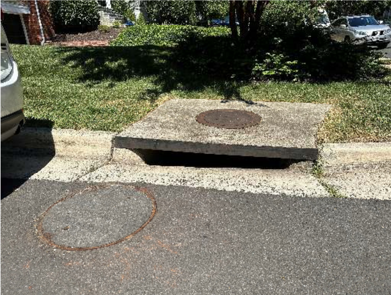
Picture 4: Storm drain curb inlet (007610IN), which conveys flow from Dogwood Drive and ultimately drains to the eastern storm drain system along Valley Drive, facing north. Also shown, storm drain manhole 002609SMH, which flows south.
