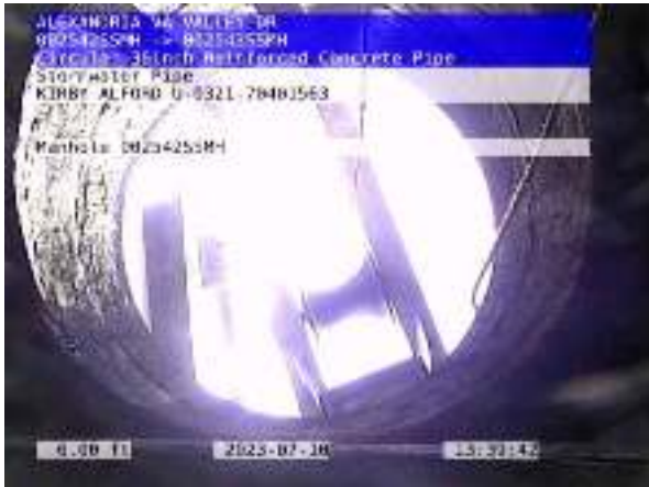
009180STMP_a32defba-bfec-48af-a515-bb31f5edad86_2023 0710_141310_579.jpg, 00:00:00, 0.00ft Manhole / 002542SSMH
