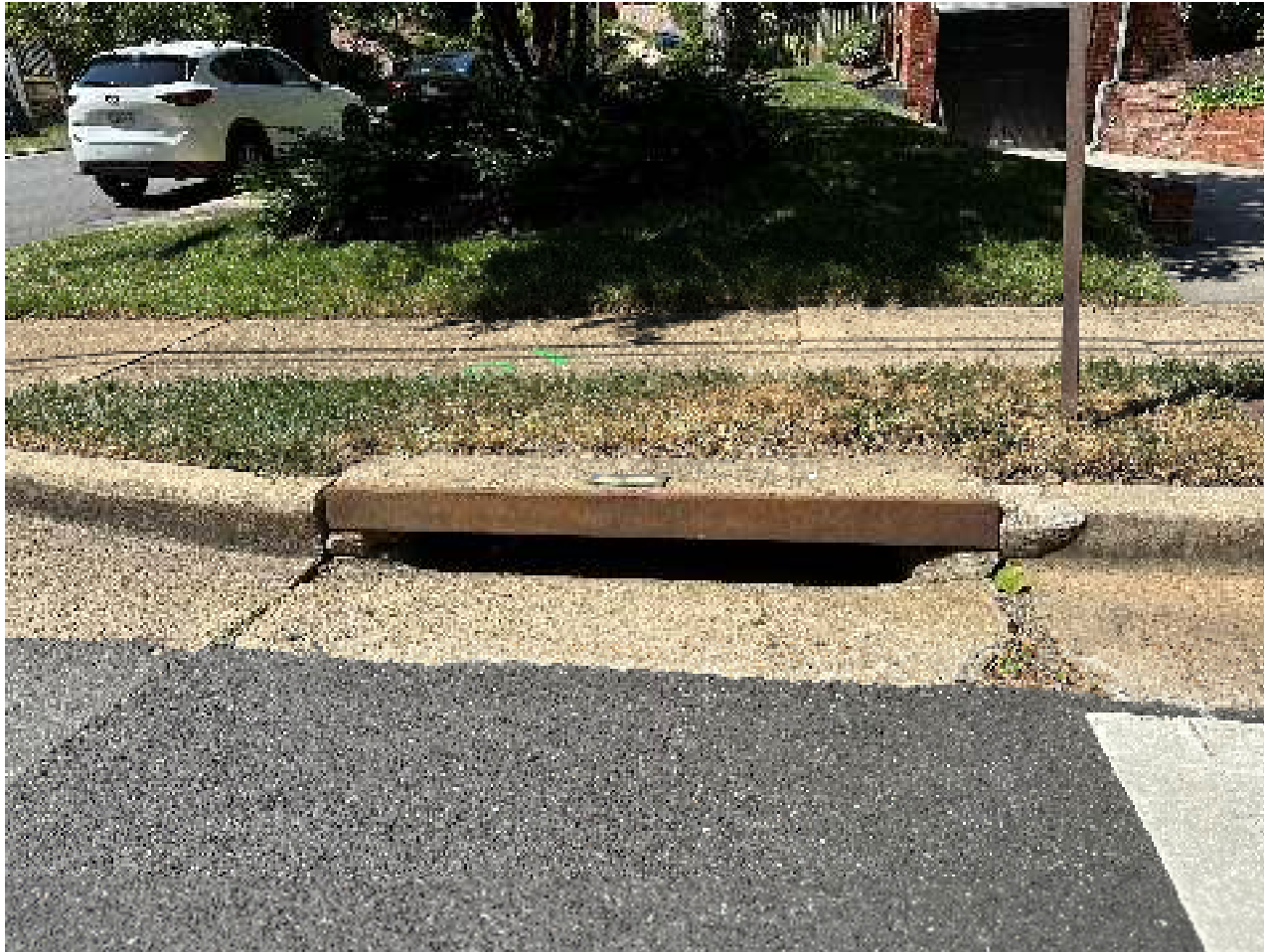
Picture 7: Curb inlet (007613IN) along the west side of Valley Drive just north of the intersection with Dogwood Drive. Approximately 5"x4', facing west.
