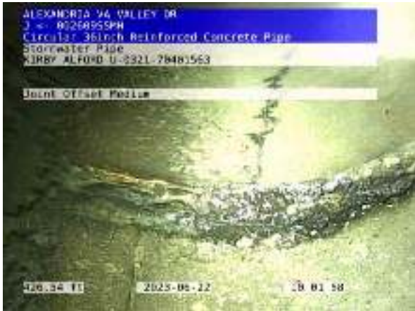
009388STMP_b6e59068-e64c-4a70-9862-1077f19174e2_20230622_103447_650.jpg, 00:09:23, 426.54ft Joint Offset Medium
