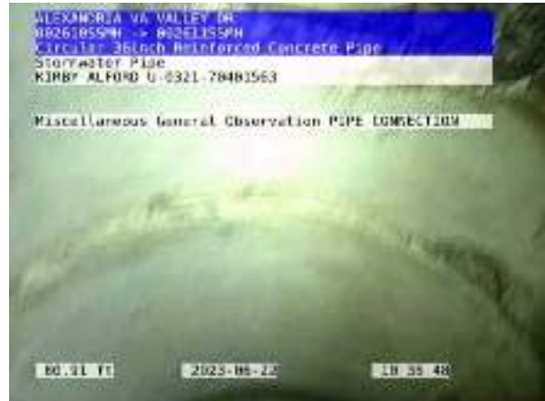
008792STMP_60e094fd-95a0-4cb6-bb58-23a85f3c91bb_20230622_110838_513.jpg, 00:01:52, 80.91ft Miscellaneous General Observation / PIPE CONNECTION
