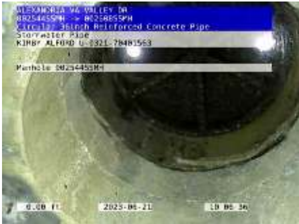
009382STMP_9d00e13b-95c5-4242-a939-e54a9e51559f_20230621_103923_945.jpg, 00:00:00, 0.00ft Manhole / 002544SSMH
