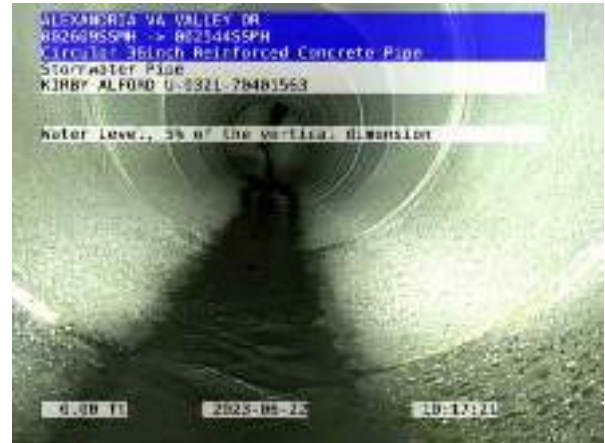
009390STMP_858fdadb-103a-4482-867f-2b2e4cd205f7_2023 0622_105011_423.jpg, 00:00:17, 0.00ft Water Level, 5% of the vertical dimension
