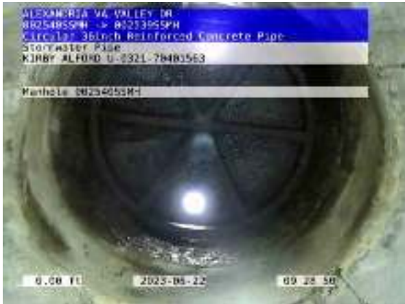
009067STMP_18122cf2-a853-43e2-977e-0a078c730dec_20230622_100139_460.jpg, 00:00:00, 0.00ft Manhole / 002540SSMH
