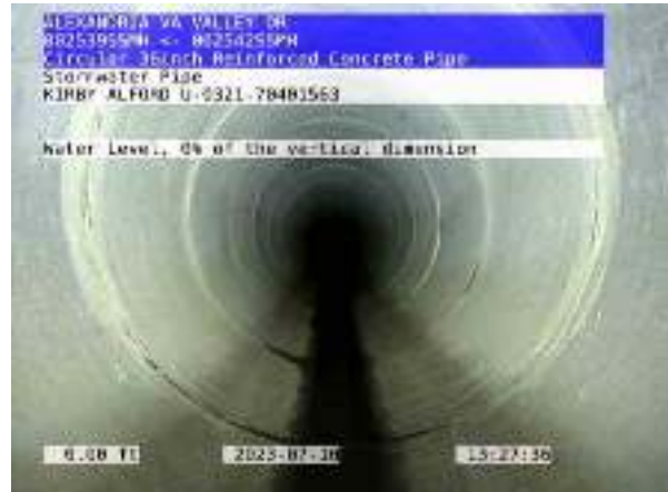
009066STMP_b347aec2-bdd4-4ef4-8183-8aa86fba86b6_20230710_140104_187.jpg, 00:00:19, 0.00ft Water Level, 0% of the vertical dimension
