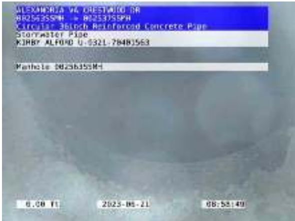
007462STMP_c3fa7375-67e8-48da-9ca1-8f9d26eca7a9_20230621_093137_224.jpg, 00:00:00, 0.00ft Manhole / 002563SSMH
