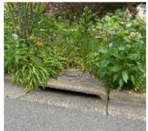
Photo 5: Curb inlet along Crestwood Drive, just west of Valley Drive
