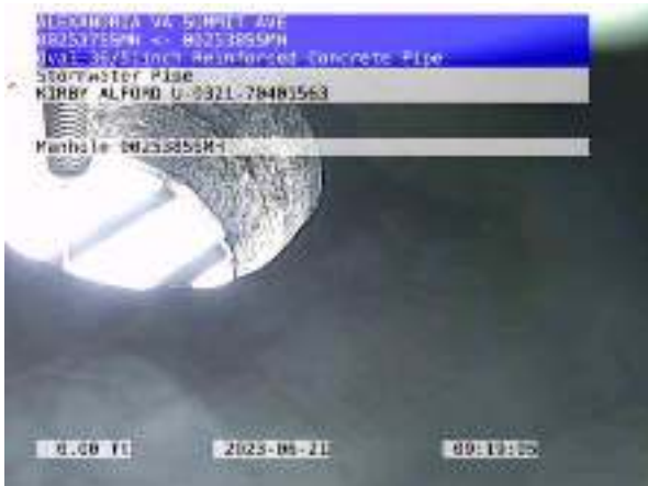
014918STMP_16507180-60fe-420d-8f5a-d67034a7c50a_20230621_095153_105.jpg, 00:00:00, 0.00ft Manhole / 002538SSMH
