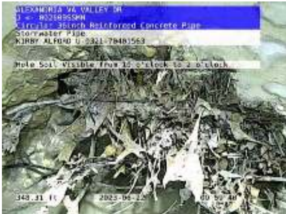
009388STMP_dc43dbdf-9e14-404f-a375-10f772fded3d_20230622_103229_549.jpg, 00:07:31, 348.31ft Hole Soil Visible from 10 o'clock to 2 o'clock
