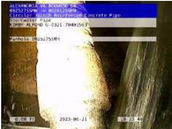
009389STMP_ece1cef7-738b-4e99-aaef-8660fadb2451_2023 0621_105635_970.jpg, 00:00:00, 0.00ft Manhole / 002527SSMH
