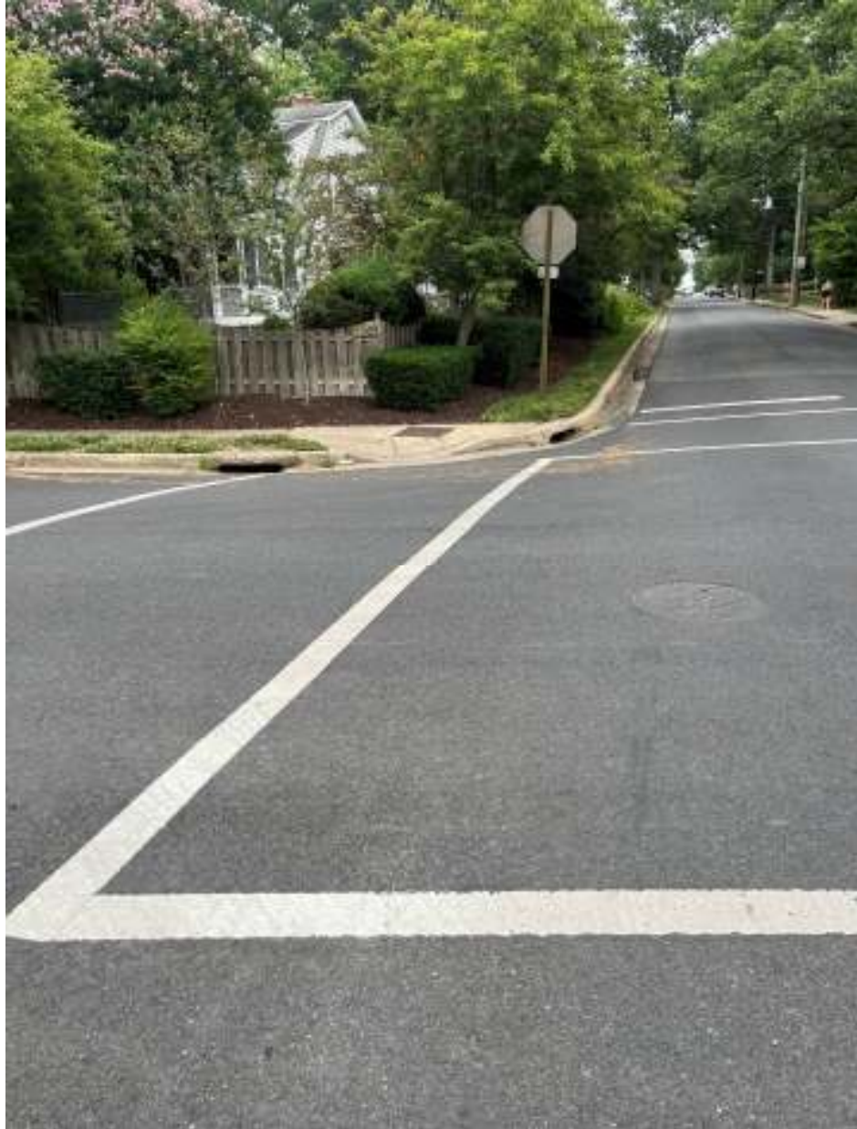
Picture 2 : Storm drain curb inlets located at the northeast corner of the intersection at Summit Avenue and Valley Drive. Facing northeast.
