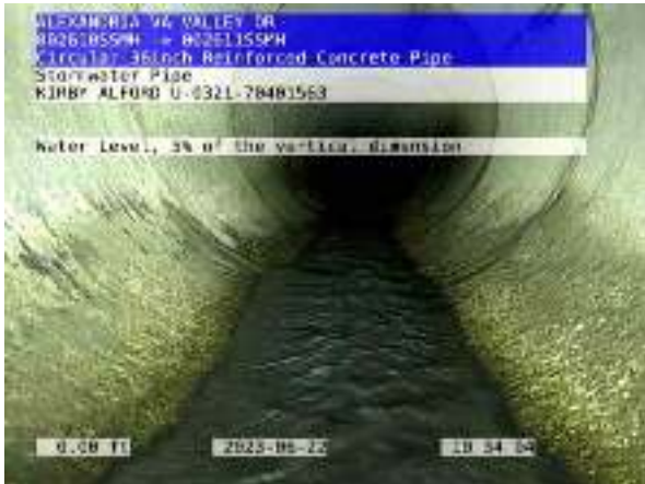
008792STMP_ad28dbee-ff13-4b32-9bac-40f9fa4c84f_20230622_110654_415.jpg, 00:00:15, 0.00ft Water Level, 5% of the vertical dimension
