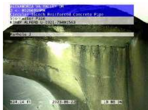
009388STMP_ddb6e932-6b05-455a-be2b-dfc3ca6f6425_20230622_104056_211.jpg, 00:15:16, 624.14ft Manhole / J
