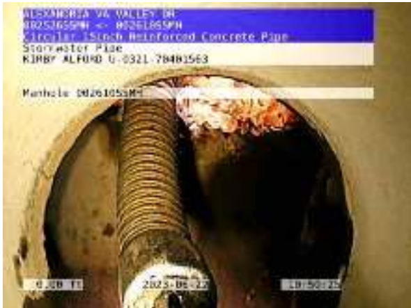
009391STMP_528e7fc8-2b98-4250-9023-dfd169812050_20230622_112314_627.jpg, 00:00:00, 0.00ft Manhole / 002610SSMH
