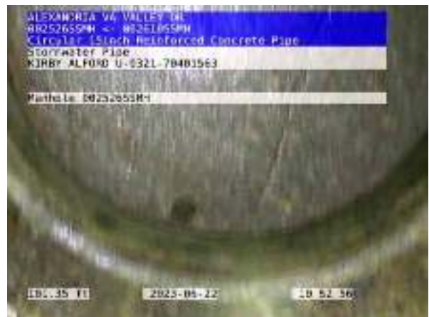
009391STMP_d9ebba60-ef8b-4d65-bc8e-d1163607f845_20230622_112546_504.jpg, 00:02:23, 101.35ft Manhole / 002526SSMH
