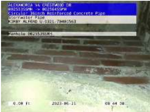
007464STMP_0701203c-0c41-4283-9004-fc5f72b1e70f_2023 0621_091655_737.jpg, 00:00:00, 0.00ft Manhole / 002553SSMH
