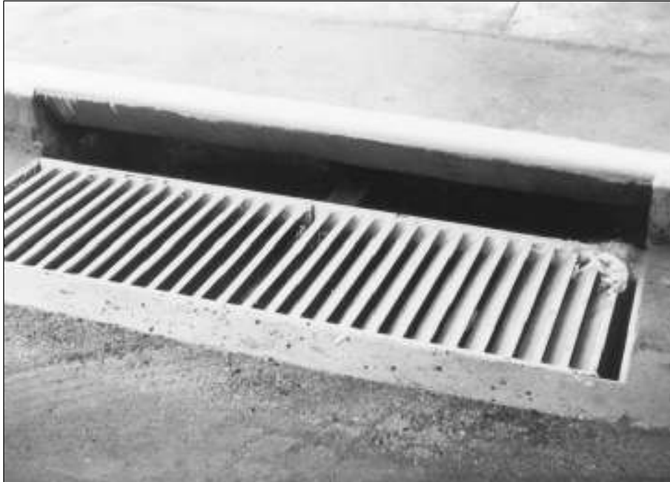
Figure 7.11. Combination curb-opening with 45-degree tilt-bar grate inlet.
