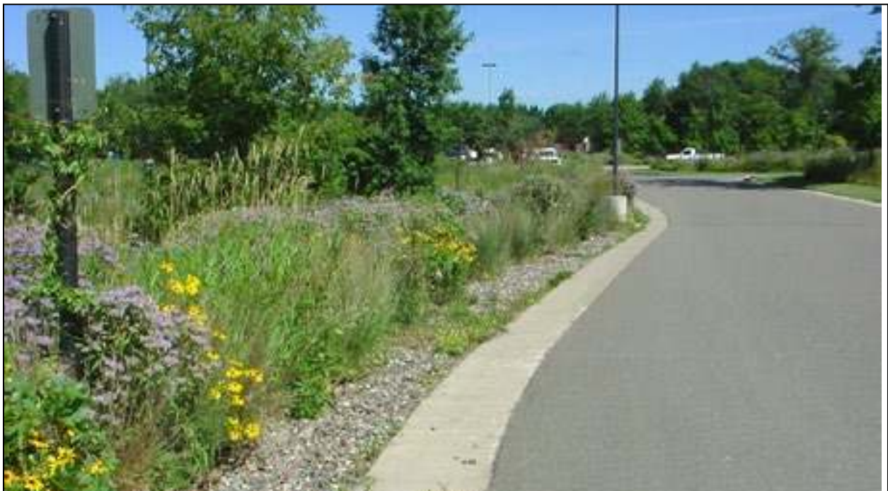
Figure 11.9. Green infrastructure practice: infiltration trench (USEPA 2021).
