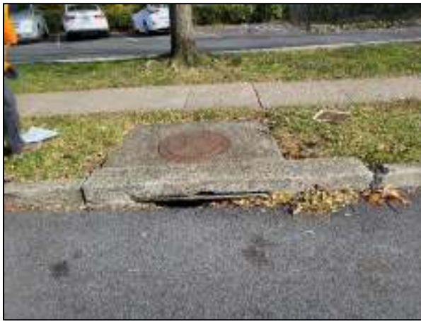
Figure 1. Curb Inlet, Valley Drive (AECOM 2022)
