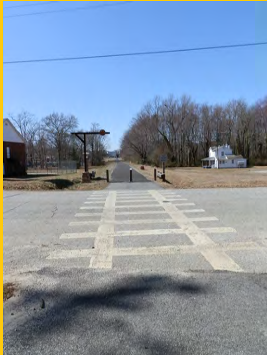
Examples of Signing and Markings for a Shared-Use Path Crossing (2009 MUTCD)
