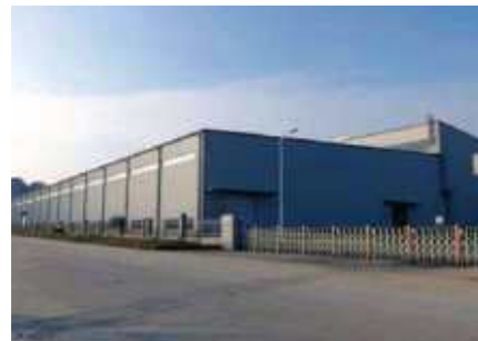
海宁玻璃厂 HAINING GLASS PLANT
