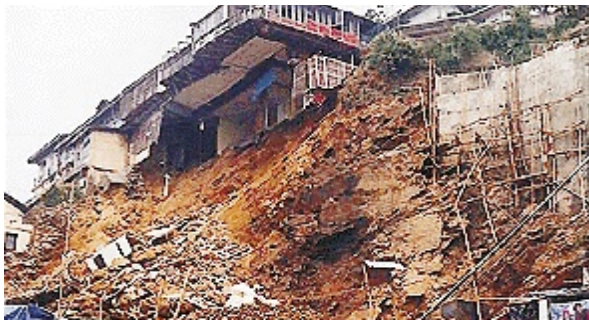
Fig 2.6.1 Landslide in hilly terrain of India
