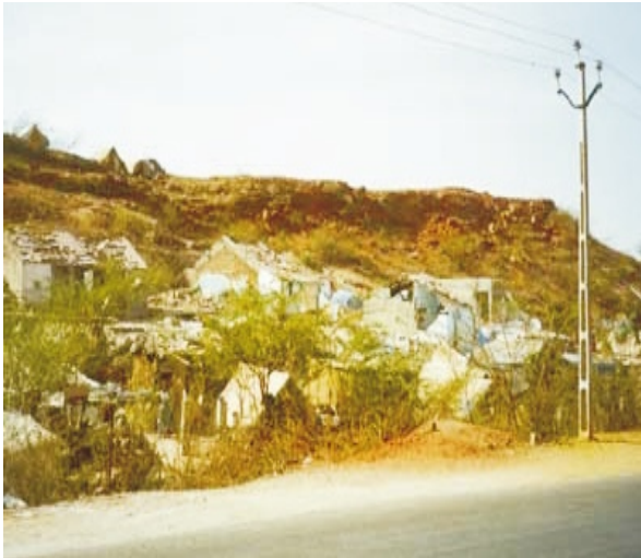
Fig 2.6.2 Bhachau Landslide - The land slipped during the 26 th January 2001 earthquake event in Bhachau. Note that people are still camped beneath. Monsoon rains could possibly wash the soil down slope.
