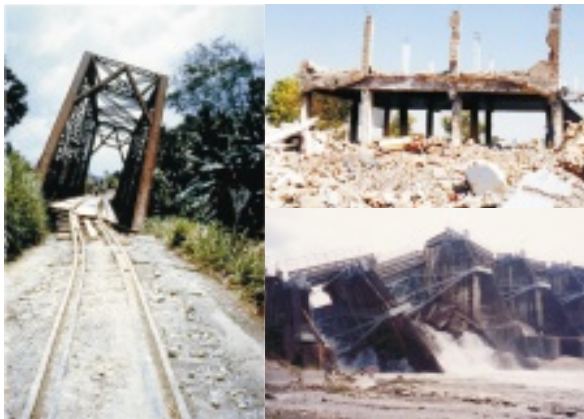
Fig 2.1.4 shows the adverse effects of an earthquake
