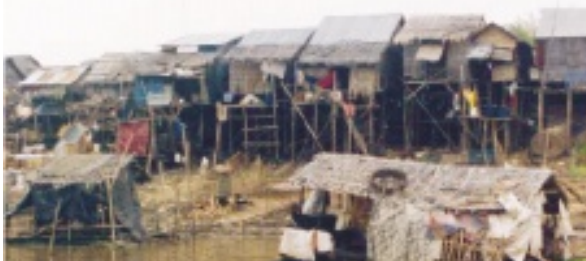
Fig 2.4.2 Houses constructed on stilts in slum areas
