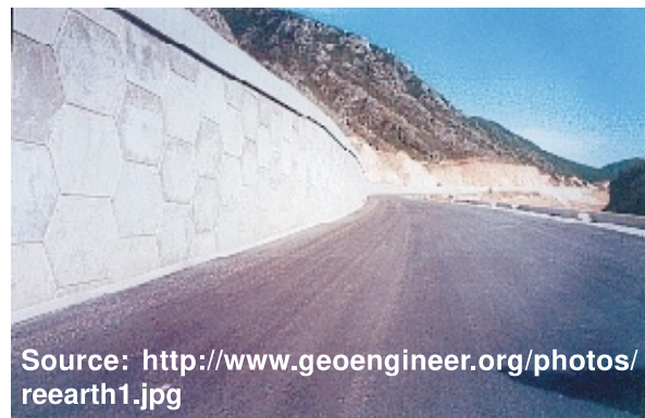
Fig. 2.6.7 Retaining wall - Reinforced wall constructed as a mitigation measure.
