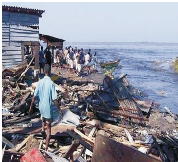
Fig 2.2.6 Damaged houses constructed on the sea coast in Chennai
