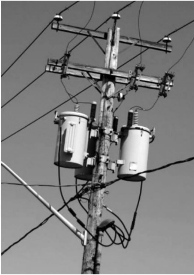
FIG. 10.3 View of a three-phase capacitor bank on a 11-kV distribution line
