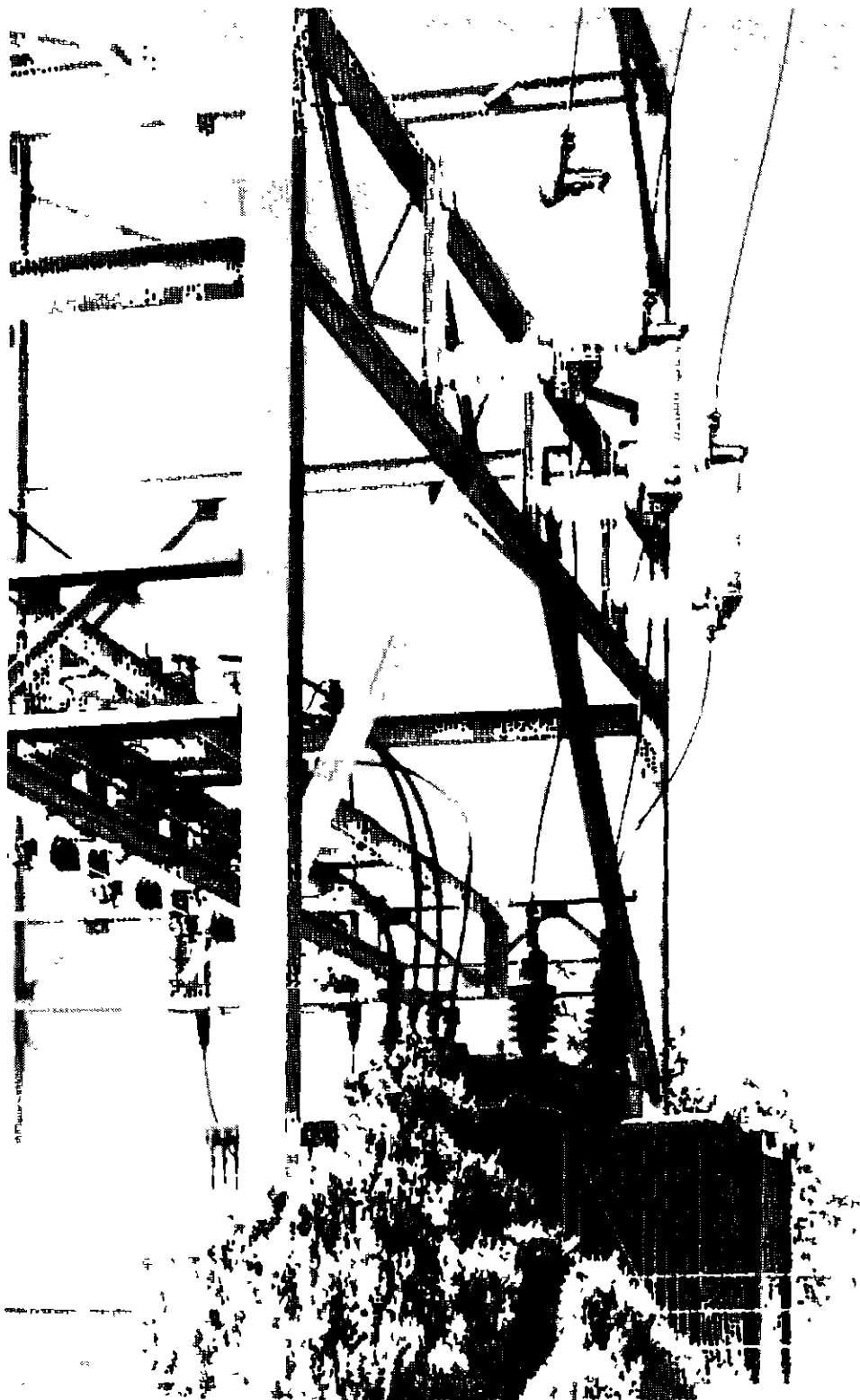
Figure 10-6 Typical transformer protection application of 34.5-kV SM-type power fuses. ( S&C Electric Company. )
