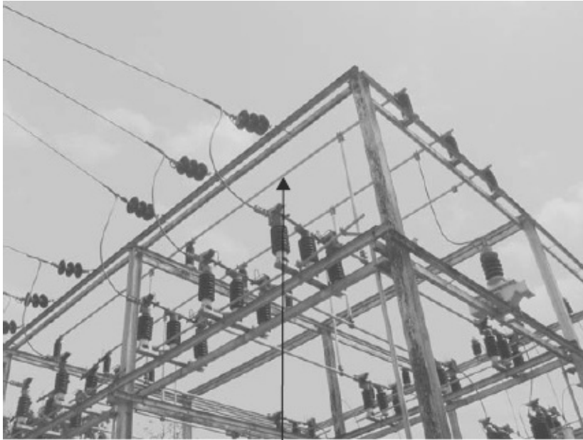
30 mm hollow aluminium bus-bar
