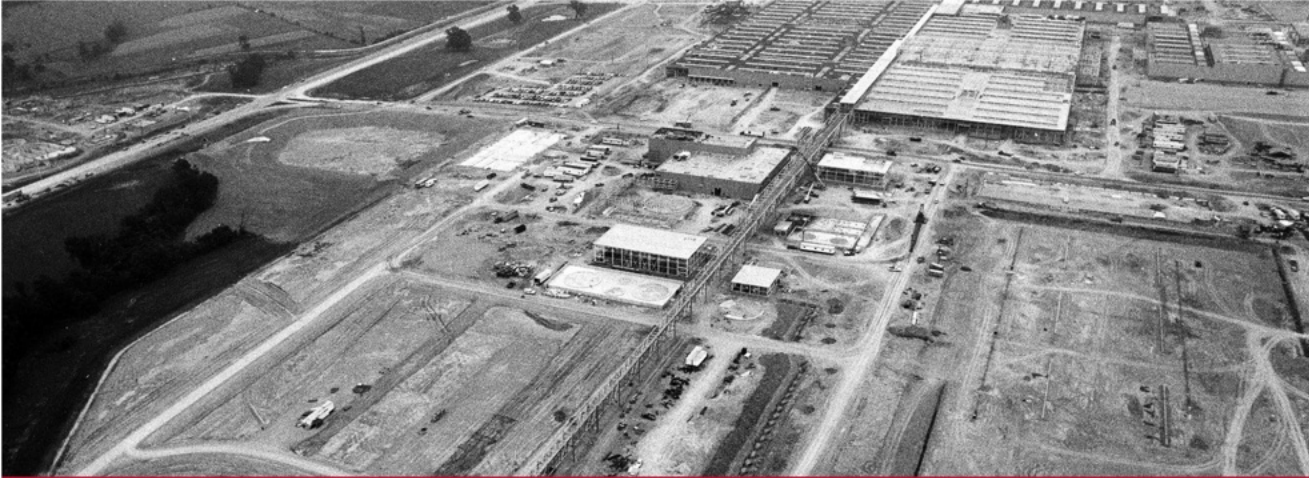
Georgetown, Kentucky under construction, May 1987
