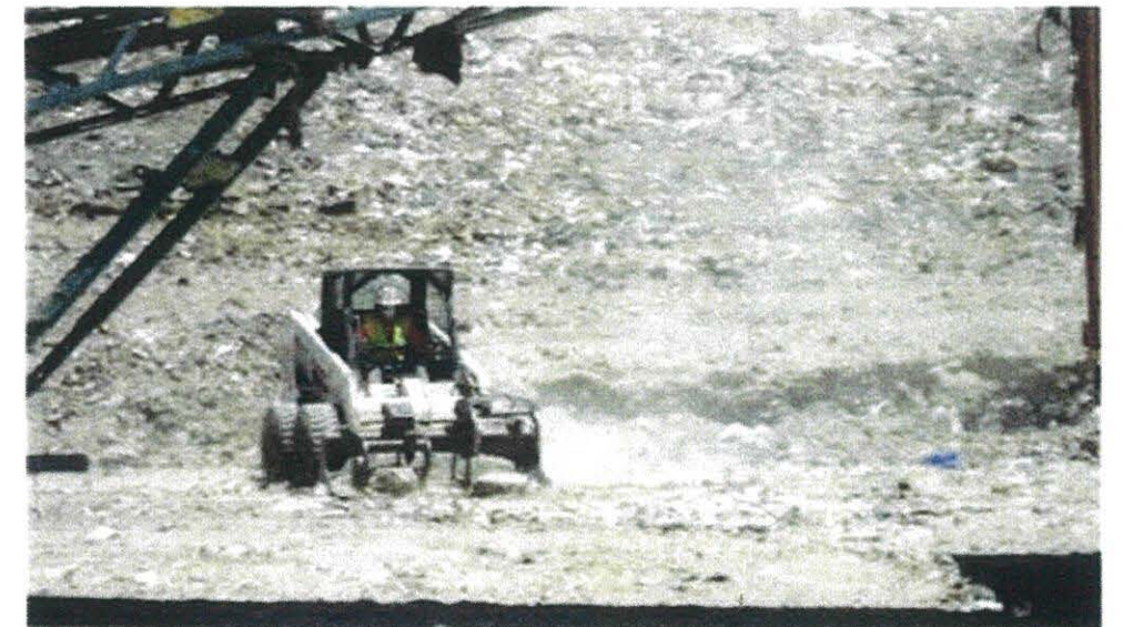
Figure 6: Use of loader for waste sorting and handling
