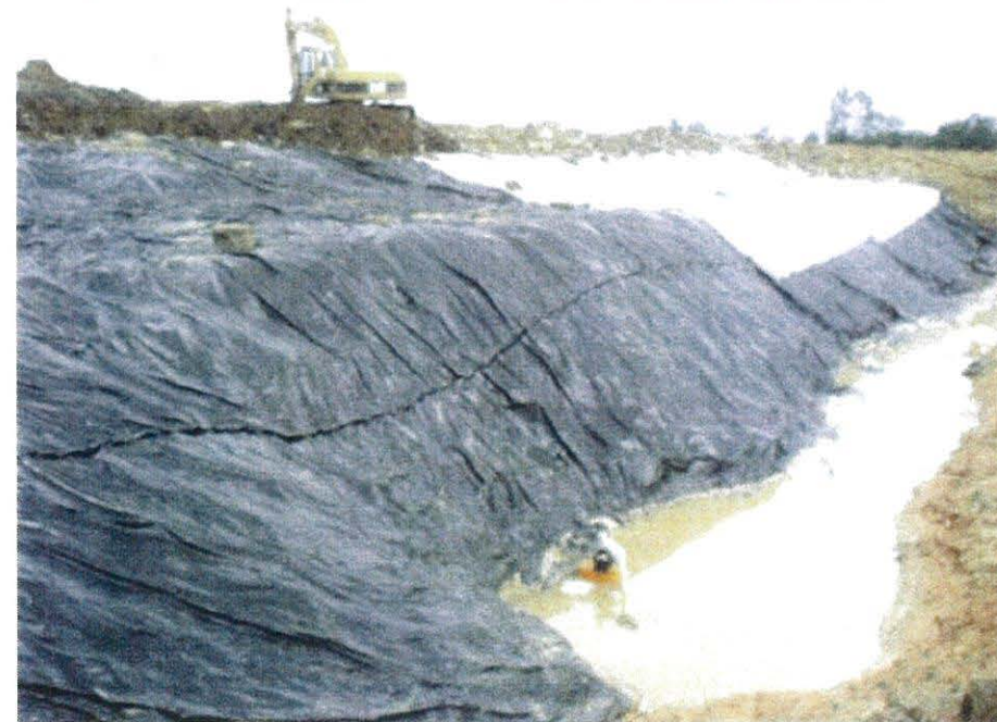
Figure 13: Use of Geomembrane/HDPE liner for daily cover
