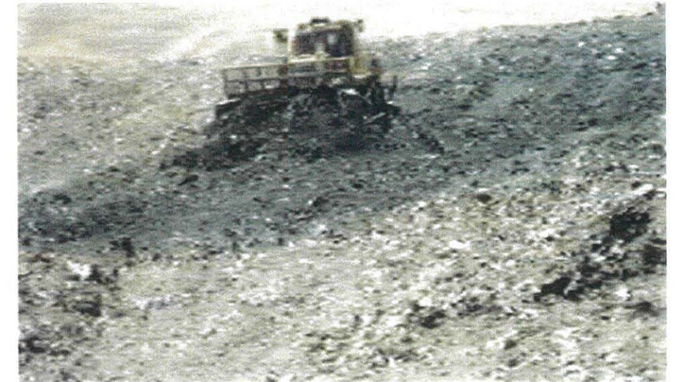
Figure 5: Landfill mining methods - Waste Scraping
