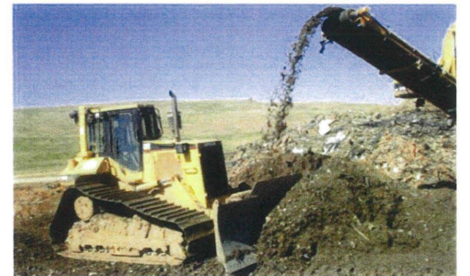
Figure 11: Movement and stockpiling of the reclaimed soil
