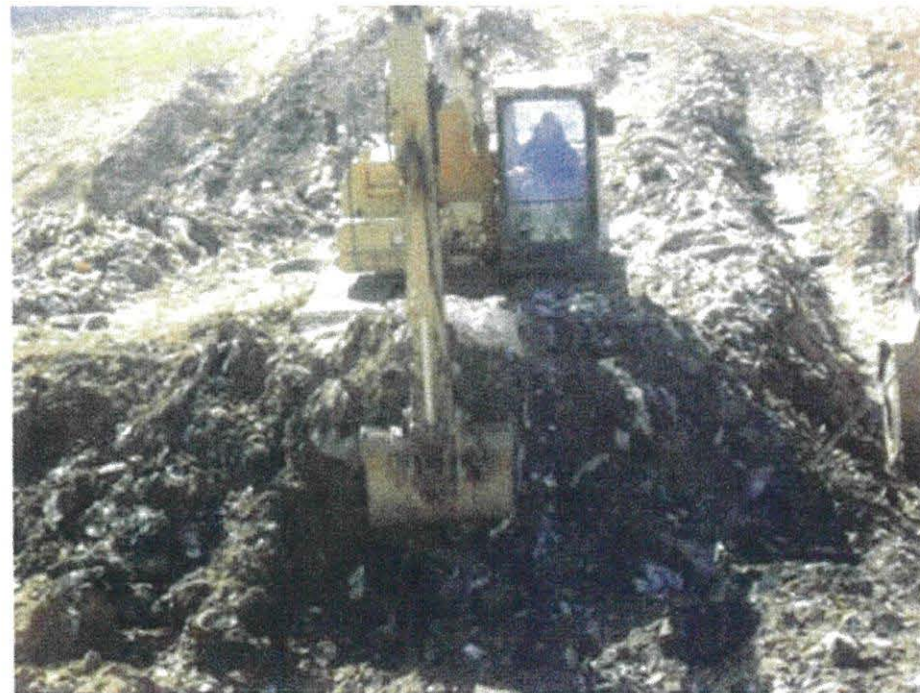
Figure 4: Landfill mining methods - Waste Excavation
