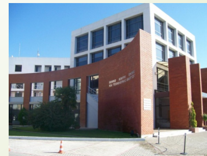
CERTH Main Building
