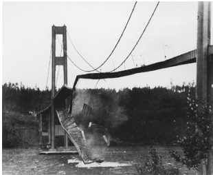
'Tacoma-narrows-bridge-collapse.jpg' see 'ATTRIBUTION'
