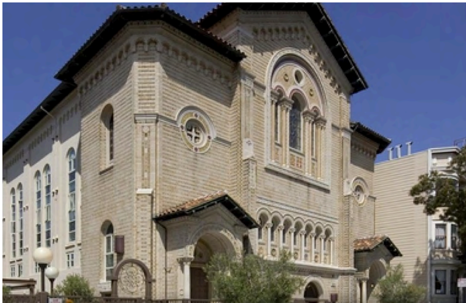
Buena Vista Terrace : San Francisco, four stories, 42 units within the shell of former Christian Sci. church. Note treatment of tall windows.
