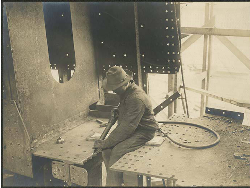
Photo: Curtis & Romans — Public domain — via Wikimedia Commons (Moran_Brothers_employee_operating_a_compressed_air_chipping_gun_Seattle_circa_1902_(MOHAI_8911).jpg)
