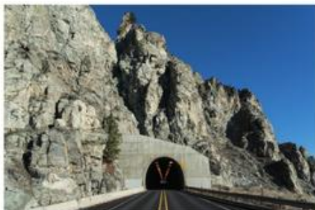
▲ Figure 20.24 Traffic passes easily through a road tunnel under a mountain.
