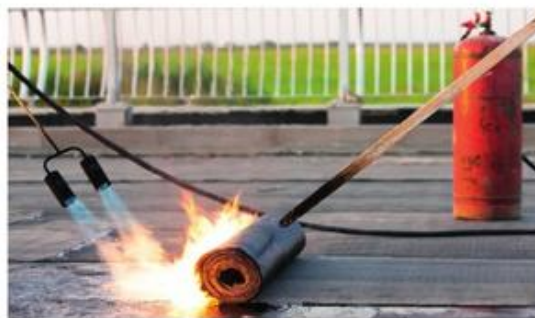
▲ Figure 23.8 Bitumen is used in road construction.
