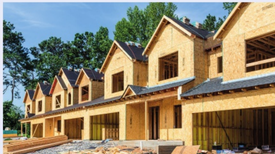
▲ Construction of new houses can be slow
