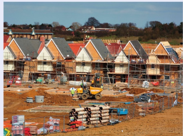
▲ Construction at a building site
