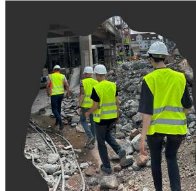
IMG 15: the team visiting the 42 construction site
