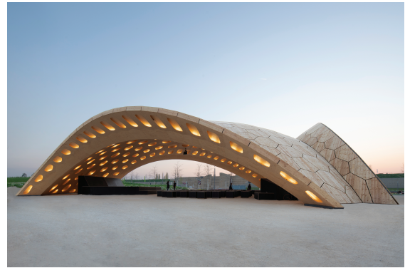
(b) The Wood Pavilion spans 30 m over a flexible event space and is built from 376 bespoke hollow wood cassette segments. ©ICD/ITKE University of Stuttgart.
