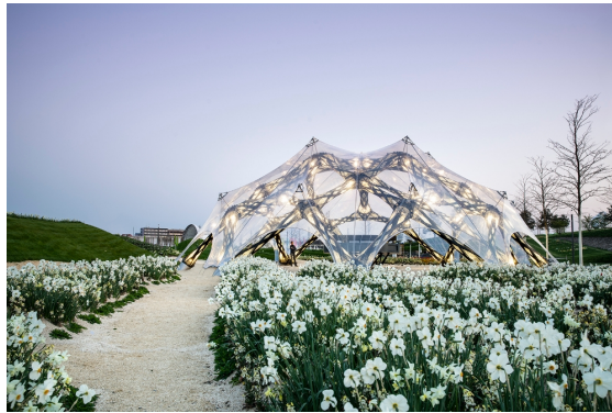
(a) The Fiber Pavilion is entirely made out of carbon and glass-fiber composites. Each component was robotically fabricated using the coreless filament winding technique. ©ICD/ITKE University of Stuttgart.
