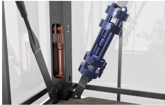
Figure 7: Rendering of actuators that are integrated into a building's support structure to compensate for the stress caused by rare, high loads.
